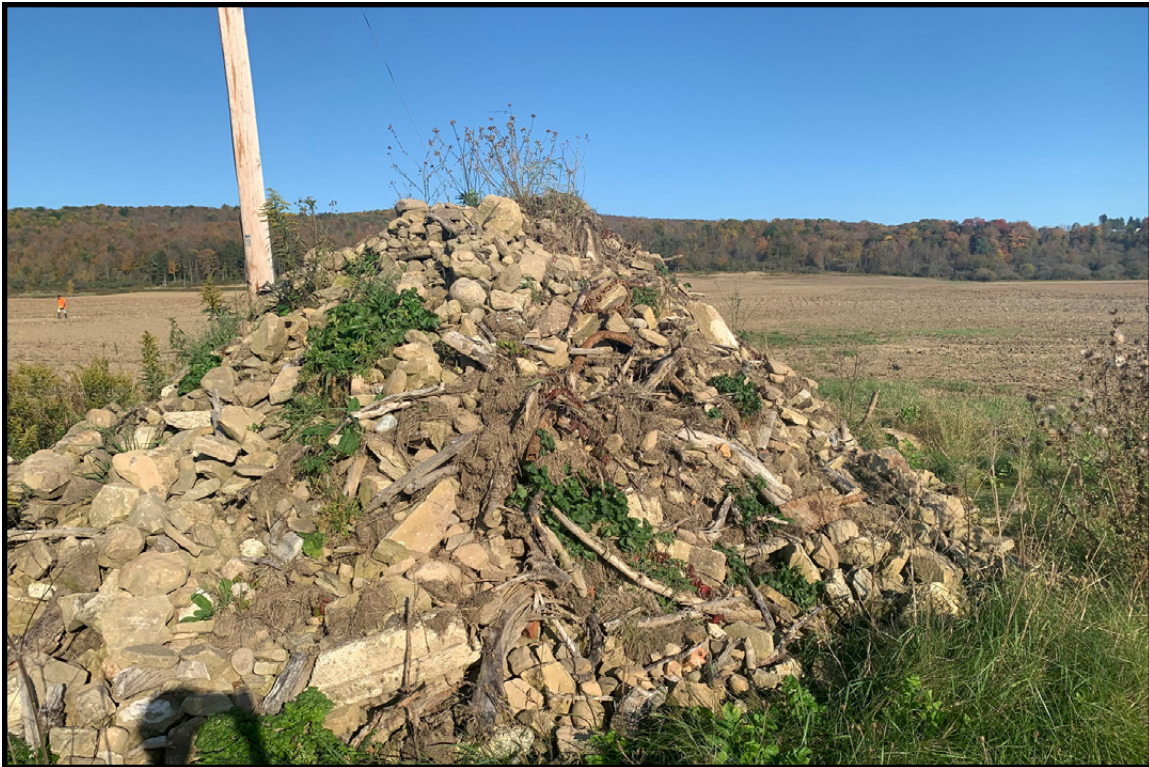
Photo 15. Facing northeast along NYS Route 16/98 showing demolition debris from the McCaa Farmstead Site. According to Jason Schwab, the current landowner, the foundations of the buildings were removed with an excavator to avoid potential damage to tilling equipment.
