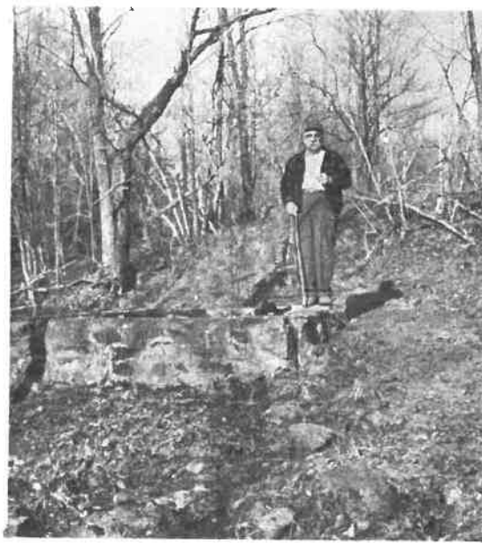
Remains of Ram on Tarbell Farm, Tarbell Hill (Enclosure)
