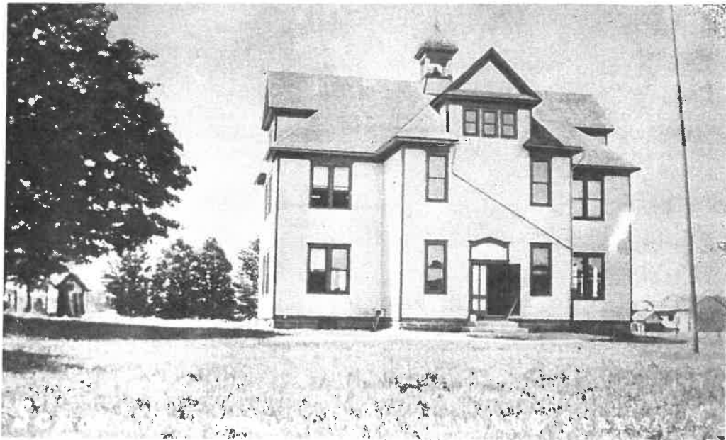
After Roof Was Raised To Accomodate More Rooms
